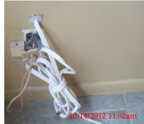
LOOSE CABLES - Loose coaxial cables need to be cut or neatly tied to abate trip hazards.
