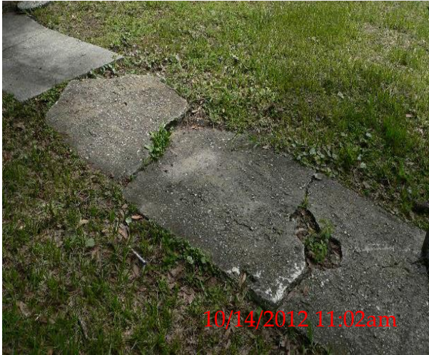
WALKWAYS / DRIVEWAYS / STEPPING STONES - must be free of trip hazards; any elevation over 2" needs to be abated.
