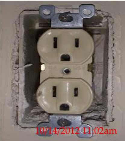
MISSING OR DAMAGED OUTLET/SWITCH COVERS - Verify all missing or damaged outlet or switch covers are replaced and covered.
