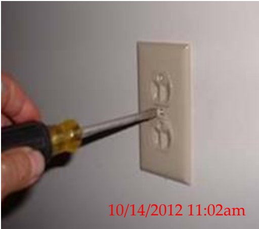
MISSING OR DAMAGED OUTLET/SWITCH COVERS - Verify all missing or damaged outlet or switch covers are replaced and covered.
