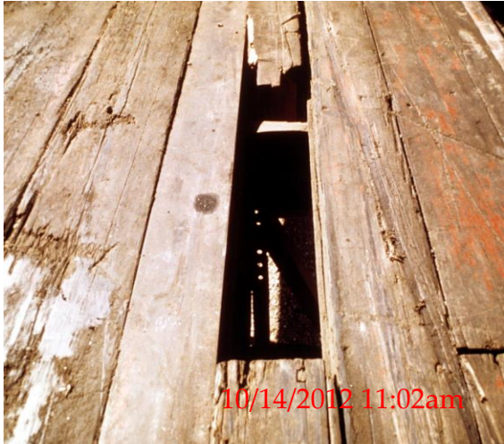
FLOOR DAMAGES - must be properly secured/repaired with plywood.
