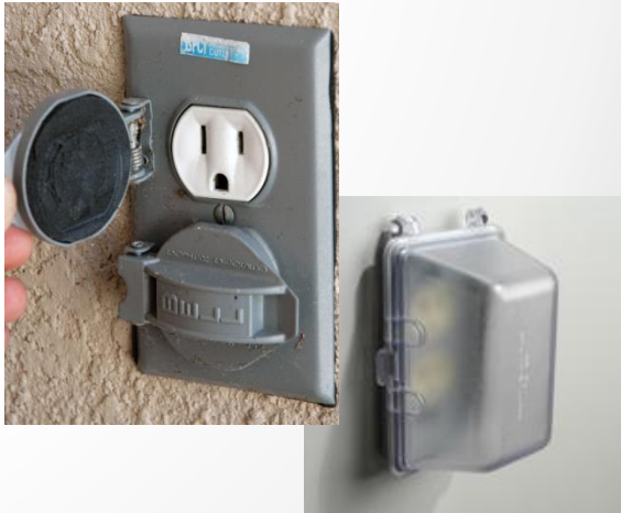
EXTERIOR OUTLET COVERS - Verify exterior outlets are covered with weather proof covers.
