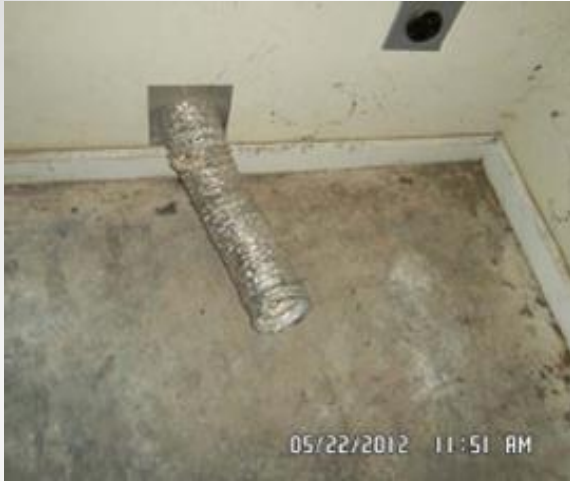
DRYER VENTS – Must be covered with cap or tape to prevent weather and/or animal intrusion.
