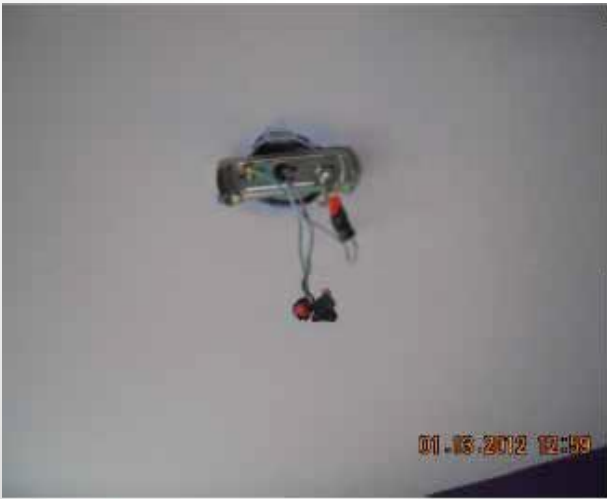
EXPOSED WIRES - Exposed wires need to be capped and taped.
