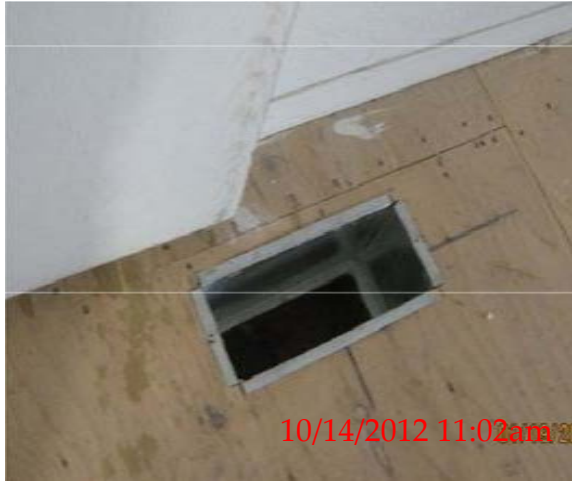
FLOOR VENTS – Must be covered with vent cover or plywood to abate trip hazards and animal intrusion.
