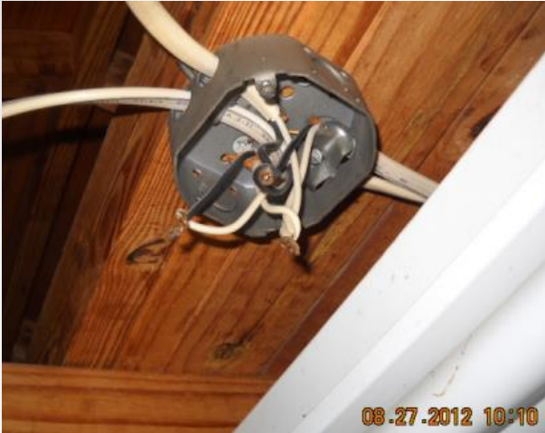
EXPOSED WIRES - Exposed wires need to be capped and taped.
