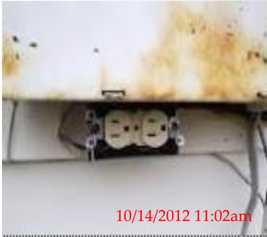
EXTERIOR OUTLET COVERS - Verify exterior outlets are covered with weather proof covers.
