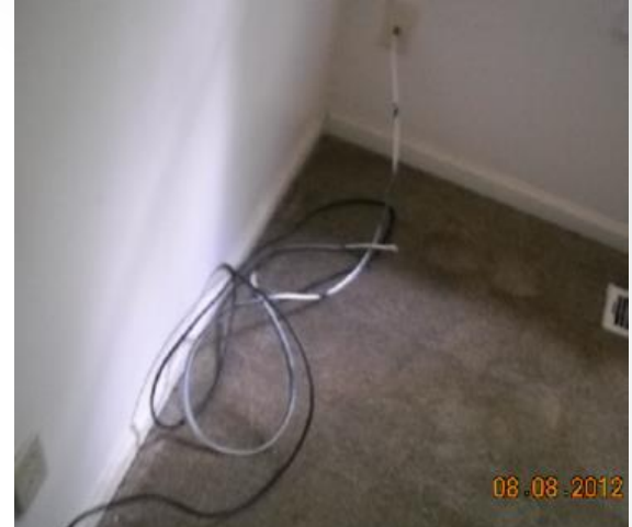
LOOSE CABLES - Loose coaxial cables need to be cut or neatly tied to abate trip hazards.
