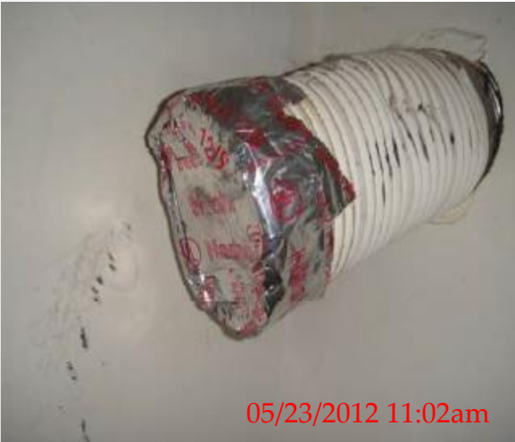
DRYER VENTS – Must be covered with cap or tape to prevent weather and/or animal intrusion.
